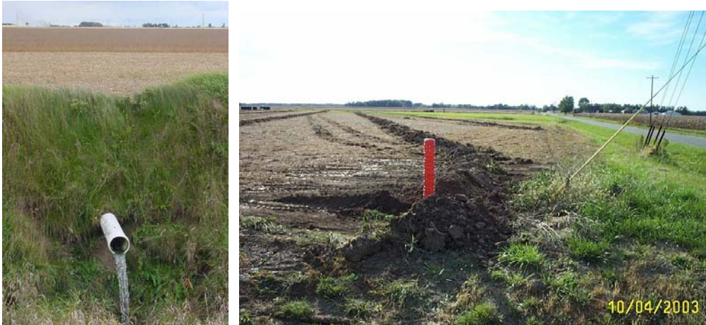
Figure 20: Tile Outlet into Drainage Ditch and Perforated Tile Riser Inlet
